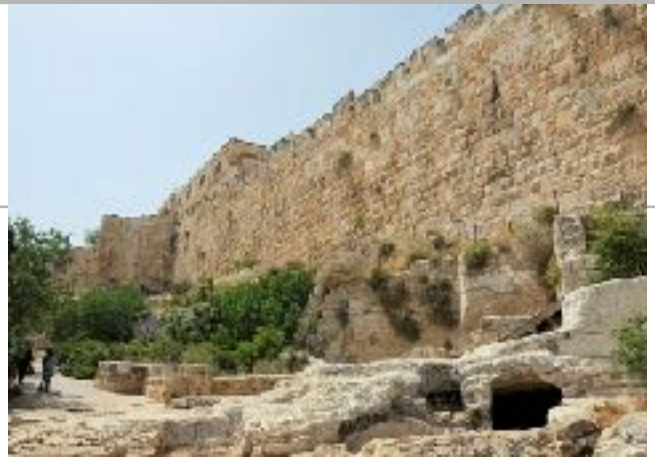
Part of the old city wall rebuilt in Nehemiah's time.
